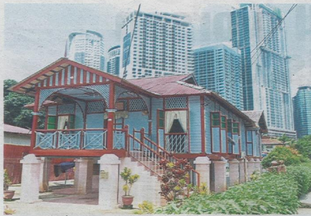
LEFT Traditional houses depicting the Malay architecture identity stand out against the backdrop of the KL city centre, giving a sharp contrast between the old and the new.
