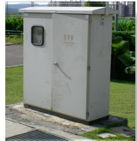
ELECTRIC FEEDER BOX
