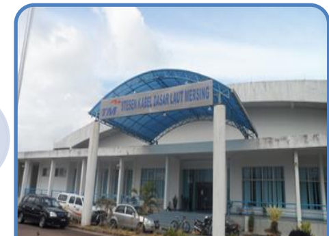
Cable Landing Station
