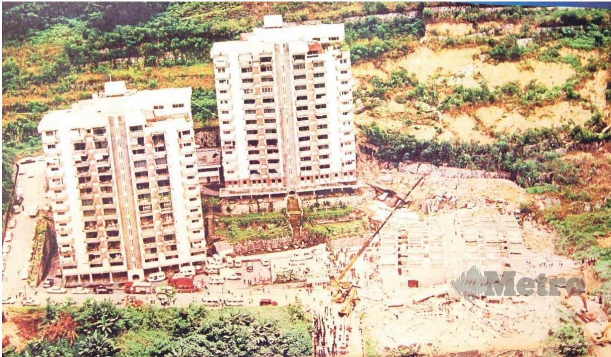
Tragedi runtuhan Kondominium Highland Tower, Bukit Antarabangsa, Ulu Klang
